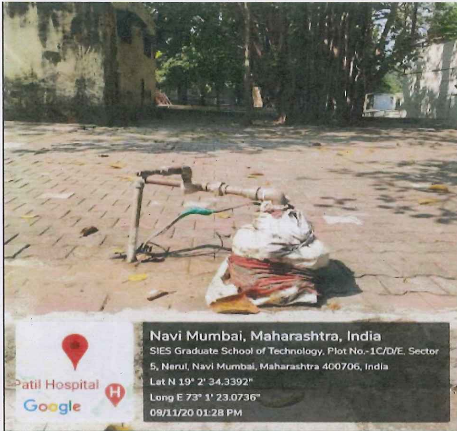
Borewell and Underground Tank
